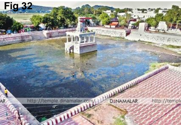
Neglected, unmaintained tanks leading to growth of weeds & breeding grounds for various diseases. Sanctity and value of temple tank and its landscape is lost
